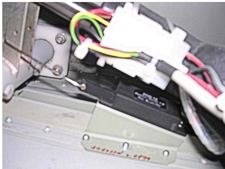
PICTURE 2 – Flaps sensor instalation
